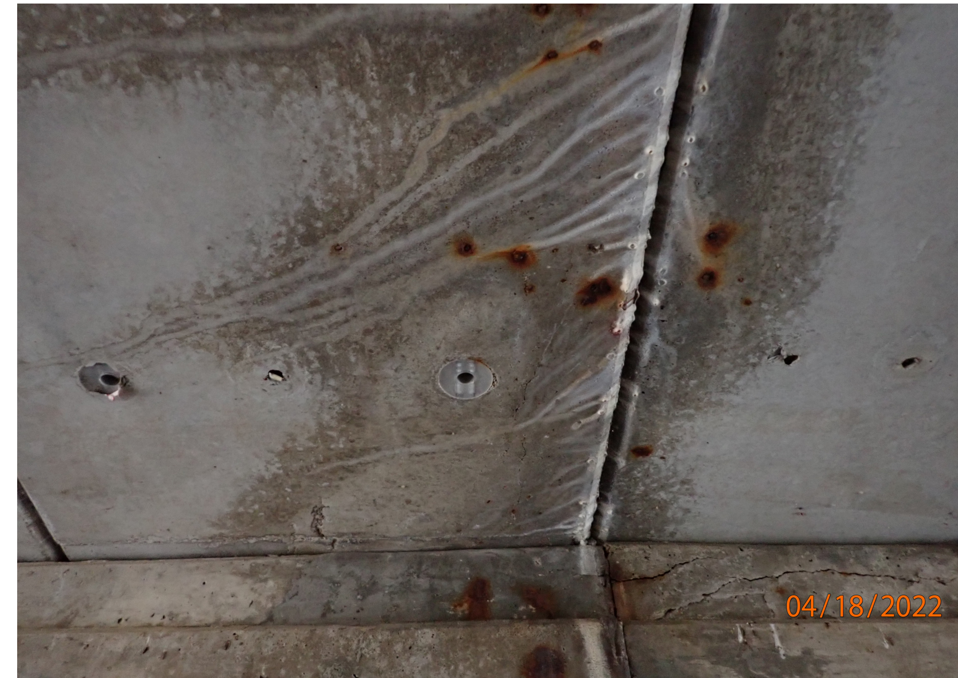
Typical Precast Prestressed Concrete beam delamination
